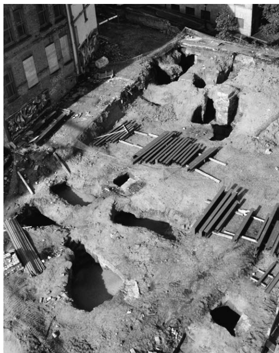
Fig. 1. A construction site in central Nottingham (seen from a tower crane) with 10 cellar caves unroofed when the ground profile was lowered by 1–2 m.
